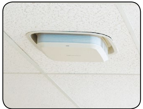
Commscope ION-E Universal Access Point
